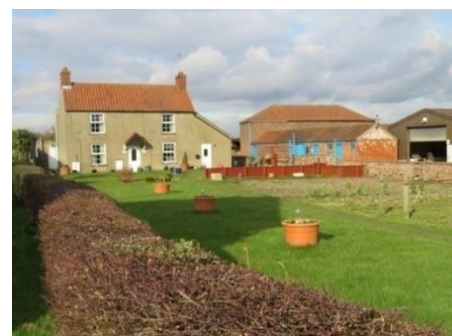
8. North End Farmhouse
