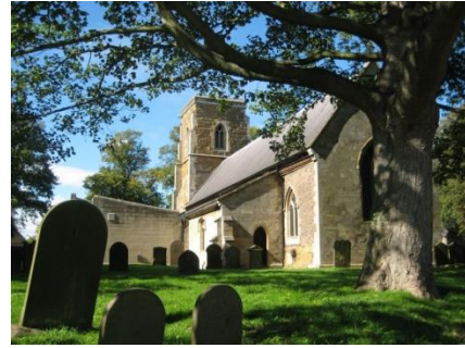
10. St Bartholomew's Church
